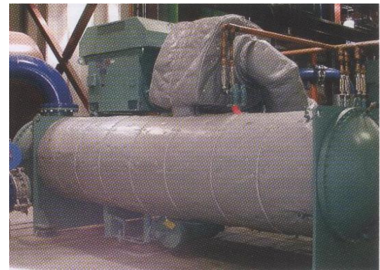
Centrifugal Liquid Chiller Design: LT250A-VP-1.5" 4 – 8 dBA Reduction
