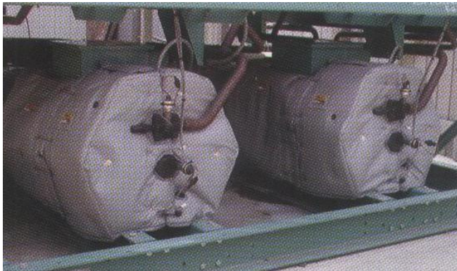
Reciprocating Compressor Enclosure Design: LT250A-VP-1.0” Thick 4 dBA Reduction
