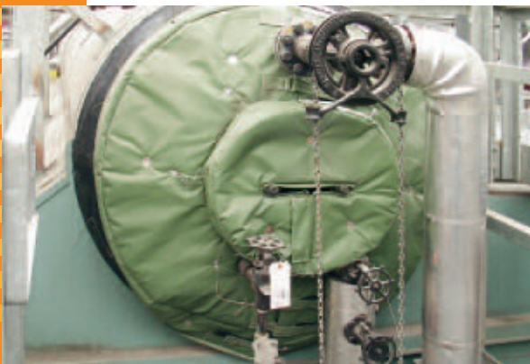
BOILER HEAD Design: Steam Drum Retrofitted with Blanket Fastener: Stainless Steel Wiretwists
