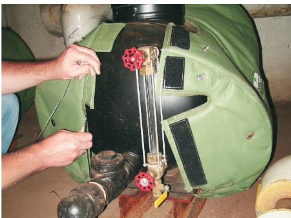
STEAM CONDENSATE PUMP & RECEIVER Design: LT450TT - 1" thickness Fastener: Stainless Steel Wiretwists and Velcro® Flaps
