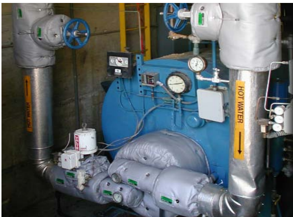
HP-HW REHEAT BOILER Exchanger Head, Valves & Fittings Design: LT450SS - 1.5" thickness Fastener: Stainless Steel Wiretwists
